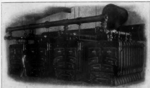
A battery of four IDEAL Sectional Steam Boilers used to warm a manufacturing plant at Buffalo, N. Y. Total capacity of battery, 28,800 square feet of radiating surface.
