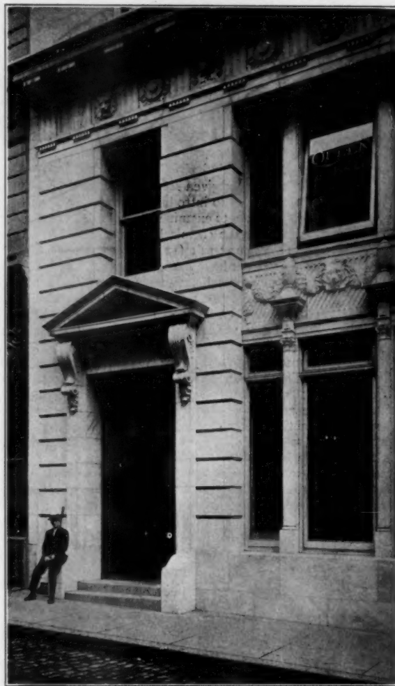
WILLIAM STREET ENTRANCE: ROYAL INSURANCE CO.'S BUILDING.
