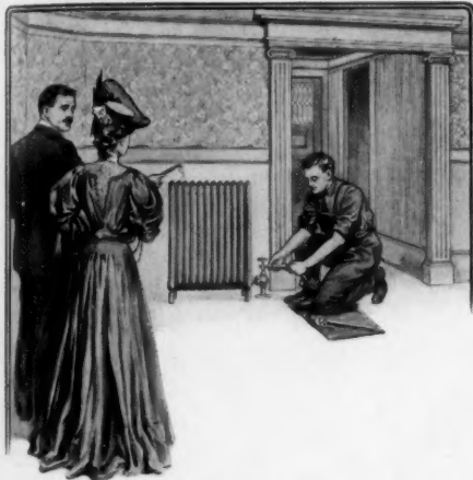
"Getting heat on" in the finishing up time
