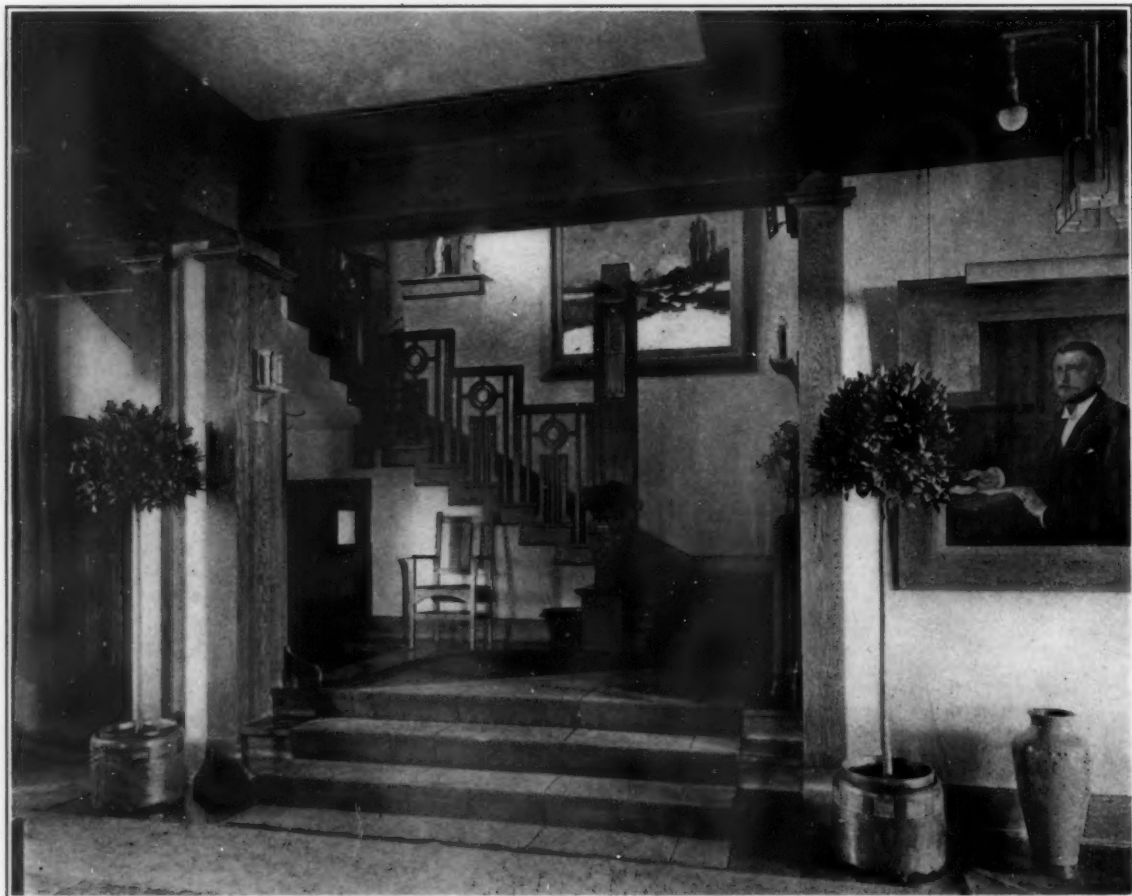
INTERIOR VIEWS: HOUSE OF HARRY RUBENS, ESQ., GLENCOE, ILL. George W. Maher, Architect.
