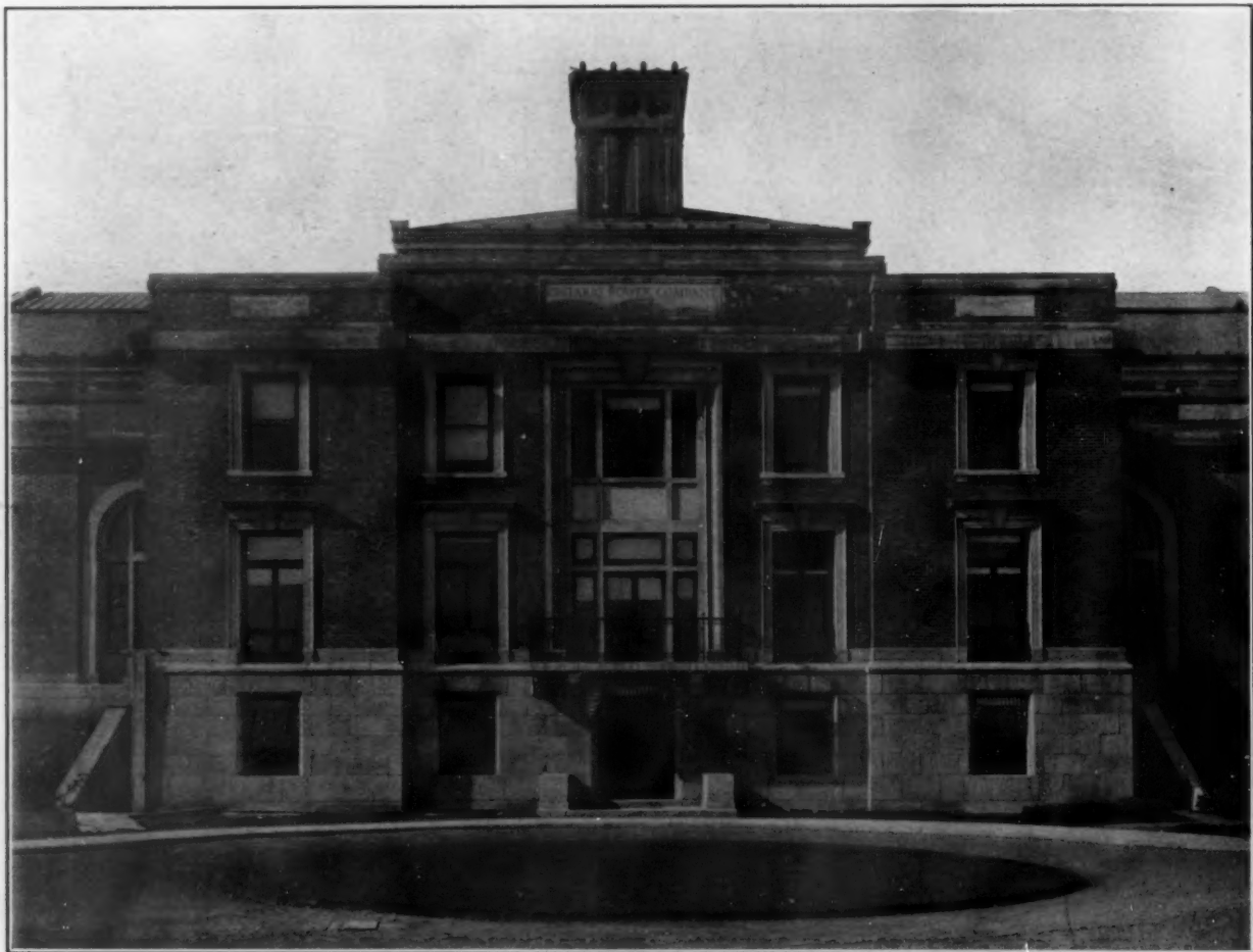
ENTRANCE DETAIL AND GENERAL VIEW, DISTRIBUTING STATION AND OFFICE BUILDING, ONTARIO POWER CO., NIAGARA FALLS, ONT., CAN.
