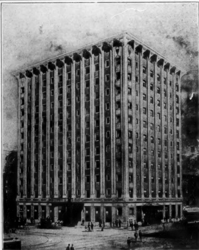
STATLER HOTEL, BUFFALO, N. Y., EISENWEIN & JOHNSON, ARCHITECTS. Built on Raymond Concrete Piles.
