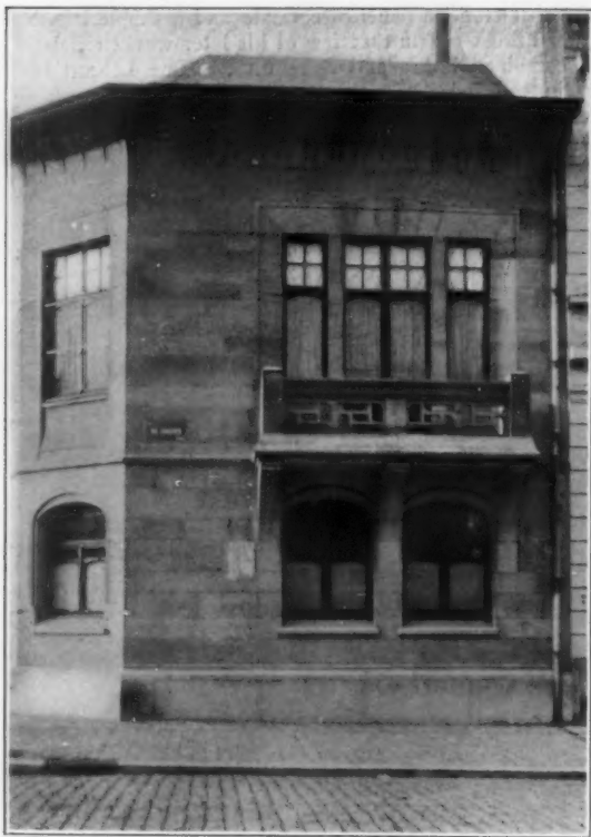
HOUSE, RUE CRAVER, BRUSSELS.
