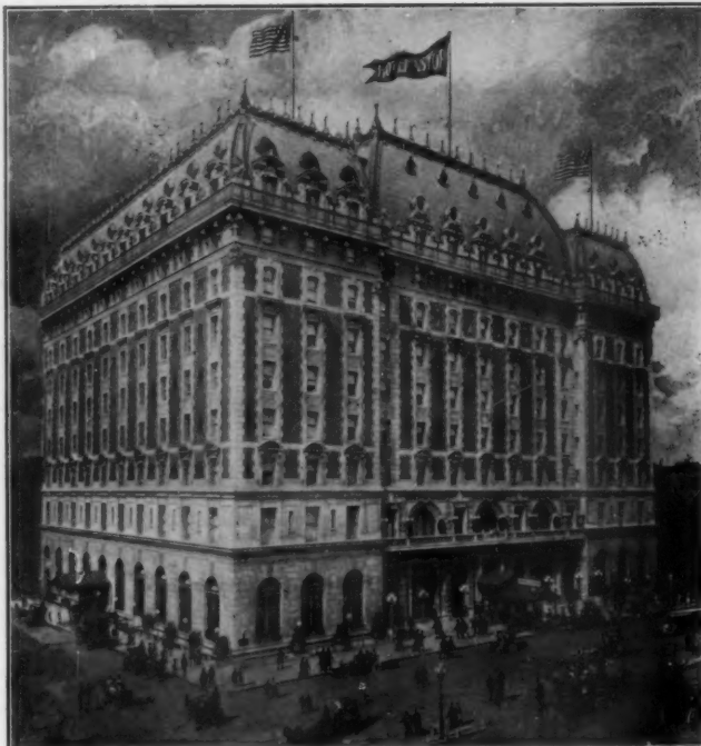
NEW ASTOR HOTEL, NEW YORK, WHERE ONE OF OUR SYSTEMS IS INSTALLED
