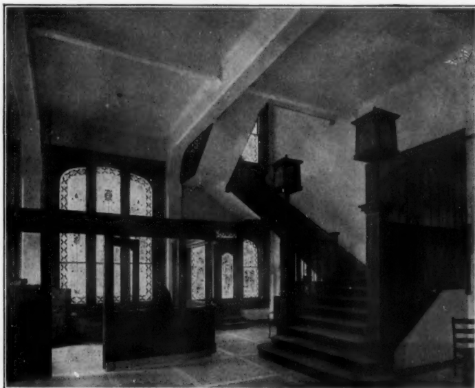
REINFORCED CONCRETE STAIRWAY Wagoner Undertaking Co., St. Louis, Mo.
