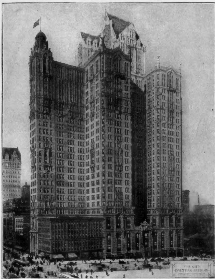
CITY INVESTING COMPANY'S BUILDING, BROADWAY AND CORTLANDT ST., N. Y. FRANCIS H. KIMBALL, Architect WEISKOPF & STERN, Engineers Rises 32 stories, 486 feet above sidewalk; cubical contents, 10,300,000 feet. WATERPROOFING, BELOW GRADE, THE HYDROLITHIC SYSTEM EXCLUSIVELY.
