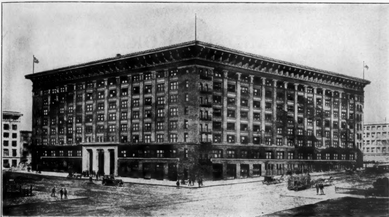
James Black Masonry & Contracting Co., St. Louis, Builders
