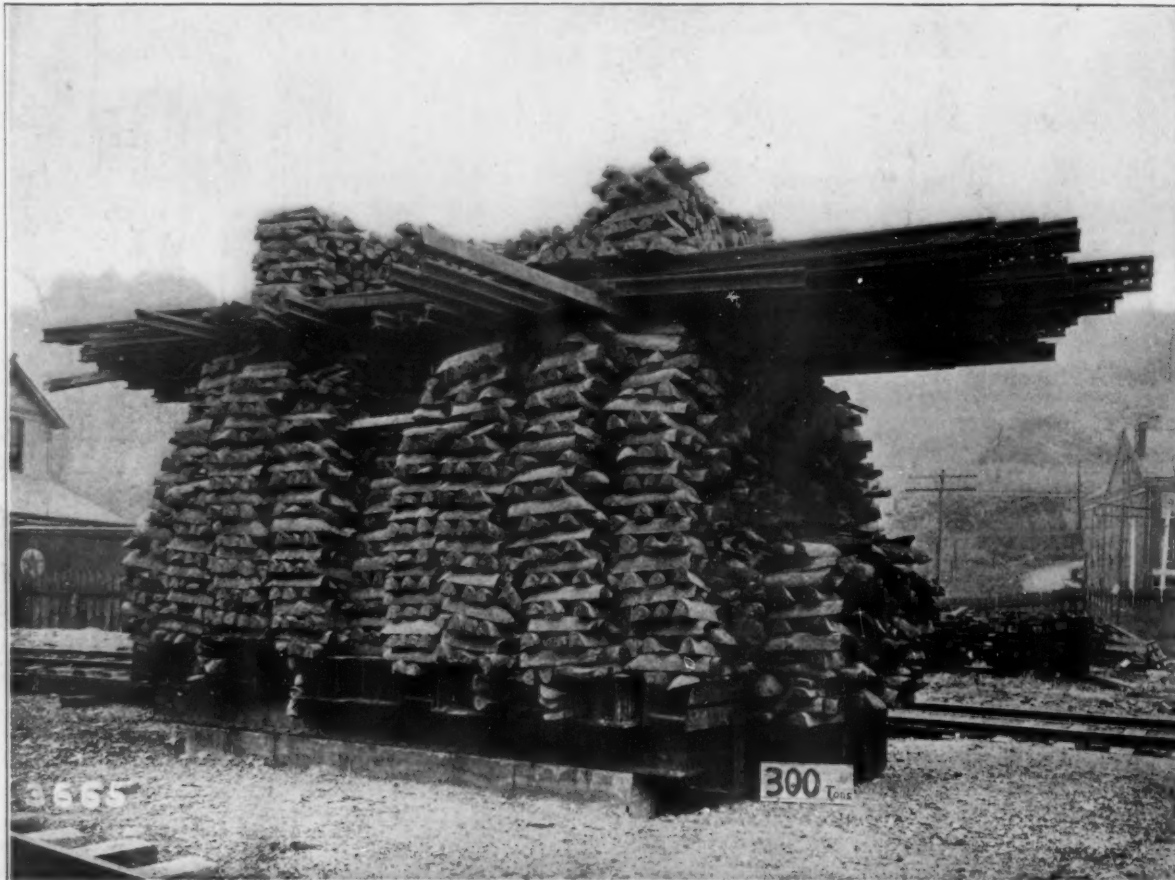
Test Load of 300 Tons on Five Sixteen-Inch Simplex Concrete Piles for Ten Days Without Any Settlement. Crane Foundations for the Westinghouse Machine Co., Pittsburg, Pa., U. S. A.
