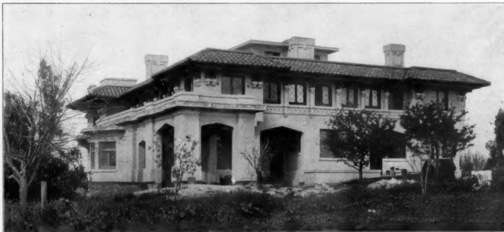
THE COMPLETED HOUSE
