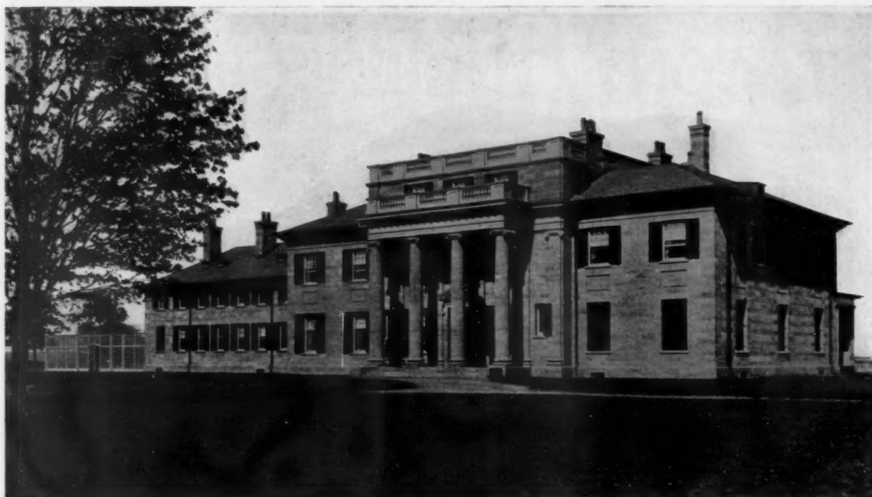
Frontispiece of January, 1907, issue of CEMENT AGE: Residence of J. R. Steers at Greenwich, Conn. Carrere and Hastings, architects. Built of hollow concrete blocks, made by dry process on machines manufactured by Noyes F. Palmer Mfg. Co., Brooklyn, N. Y.
