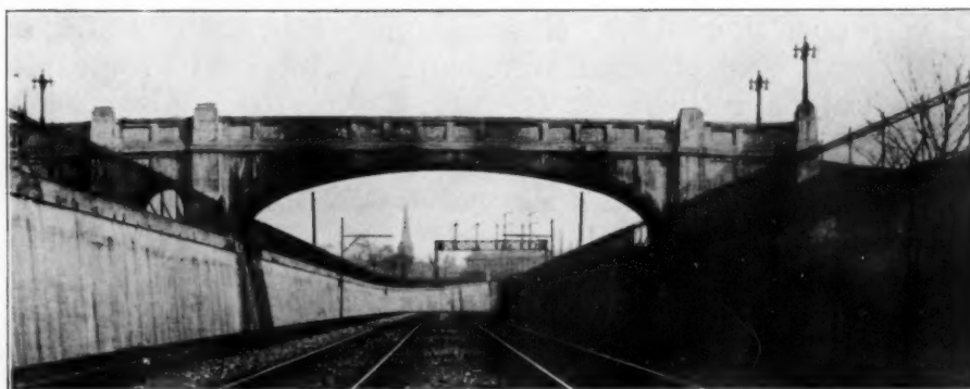
Allegheny Park Highway Bridge
