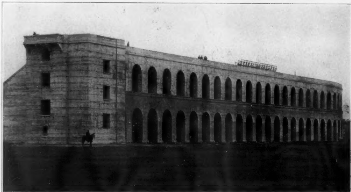
Stadium, Harvard University, built by Aberthaw Construction Co., in five and a half months
