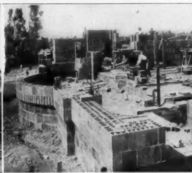
Beginning the work as viewed from the exterior
