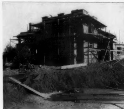
View of tile exterior walls before cement finish was applied
