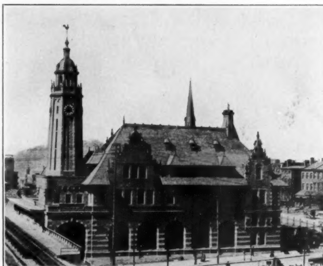
Fort Wayne Passenger Station, Pennsylvania R.R., Allegheny, Pa. Price & McLanahan, Architects All Structural Parts of Main Station, Express Building and Concourse in Hennebique System, 50 ft. Roof Trusses
