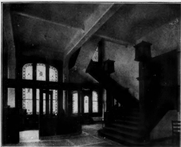
REINFORCED CONCRETE STAIRWAY
