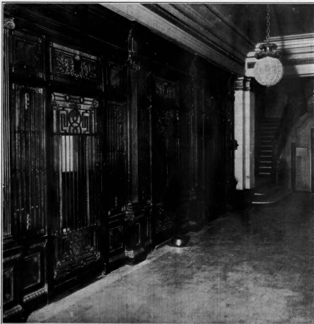
ELEVATOR ENCLOSURE, ENGINEERING SOCIETIES BUILDING, NEW YORK HALE & ROGERS and H. G. MORSE, Associated Architects
