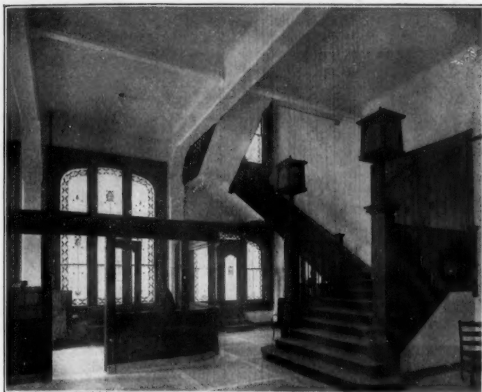
REINFORCED CONCRETE STAIRWAY
