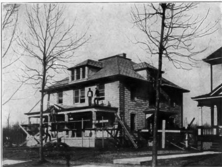
Illustrating a Concete Block House of Dr. H. C. Howard, Champaign, Illinois, Prof. F. M. White, Architect, roofed with Asbestos "Century" Shingles, laid French Method
