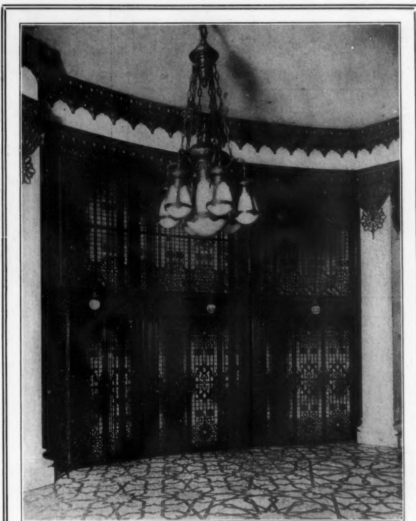
DETAIL OF ELEVATOR ENCLOSURE, ROCKEFELLER BUILDING, CLEVELAND.
