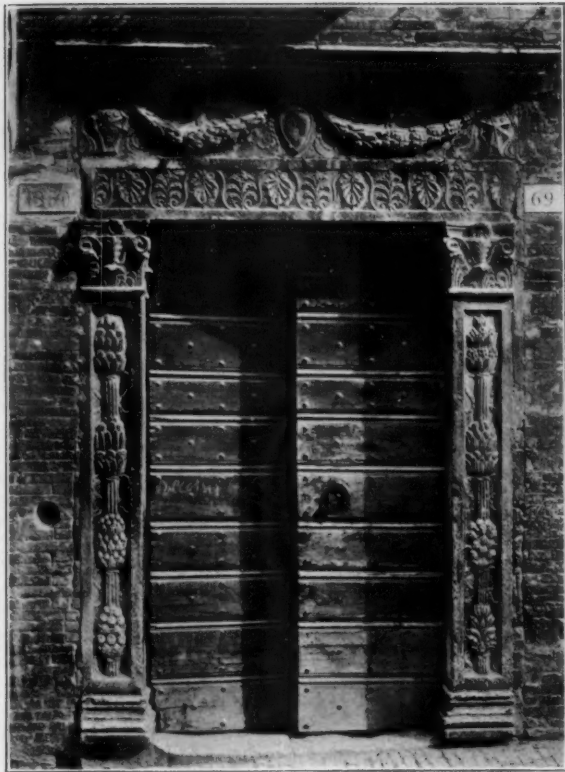
DOORWAY OF THE PALAZZO FOGLIANI, VENICE.
