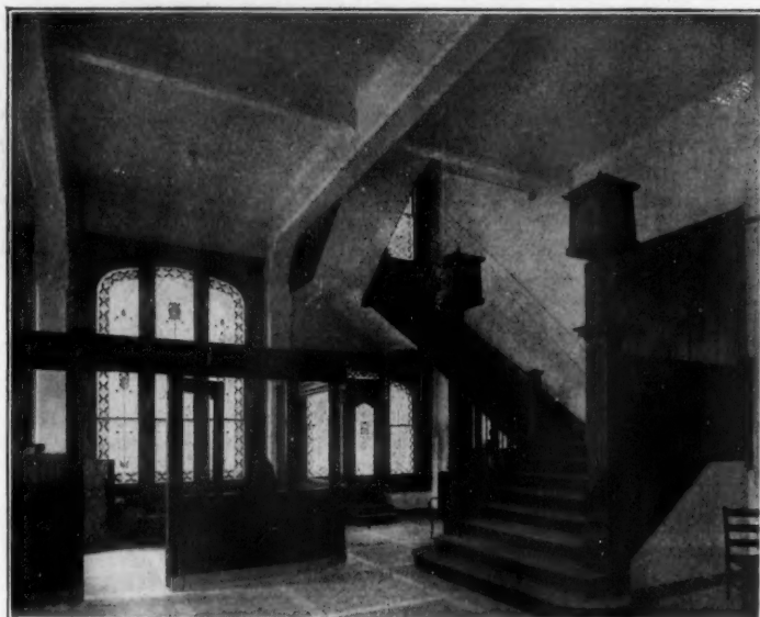
REINFORCED CONCRETE STAIRWAY
