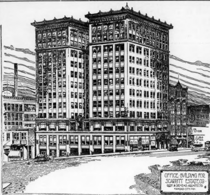
THE SCARRITT BUILDING, GRAND AVENUE AND NINTH STREETS. KANSAS CITY, MO.
