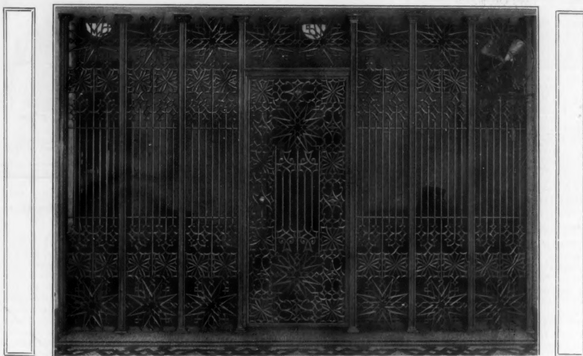
BRONZE SAFETY DEPOSIT SCREEN, SUPERIOR SAVINGS & TRUST CO., ROCKEFELLER BUILDING, CLEVELAND, OHIO. Knox & Elliott, Architects.
