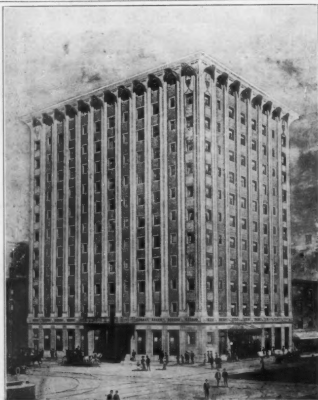
STATLER HOTEL, BUFFALO, N. Y., ESENWEIN & JOHNSON, ARCHITECTS. Built on Raymond Concrete Piles.
