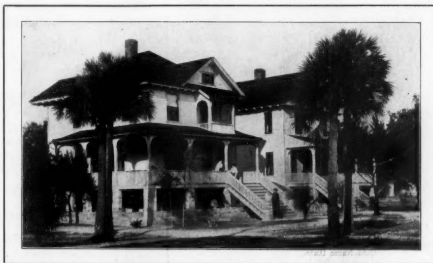
Double House at Daytona, Florida, Supplied by Kewanee Water System
