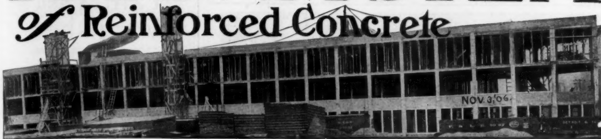
Showing Anderson Carriage Co. Factory, Detroit, in process of construction. Kahn System of Reinforced Concrete used throughout. Work completed in forty-nine days—twenty days inside contract time.
