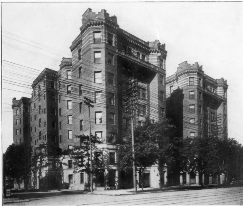
WEISSINGER-GAULBERT APARTMENT BUILDING, LOUISVILLE, KY., McDONALD & SHEBLESSY, ARCHITECTS. C. R. WATTS & CO., ENGINEERS. SUPPLIED WITH WATER THROUGHOUT BY KEWANEE SYSTEM.
