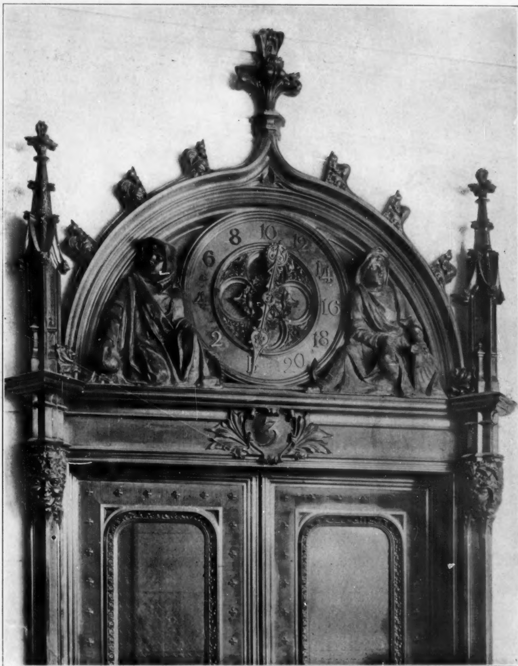
Detail of Bronze Elevator Enclosure: Trinity Building, New York.
