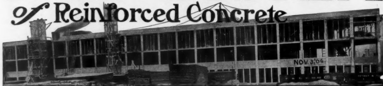
Showing Anderson Carriage Co. Factory, Detroit, in process of construction. Kahn System of Reinforced Concrete used throughout. Work completed in forty-nine days—twenty days inside contract time.
