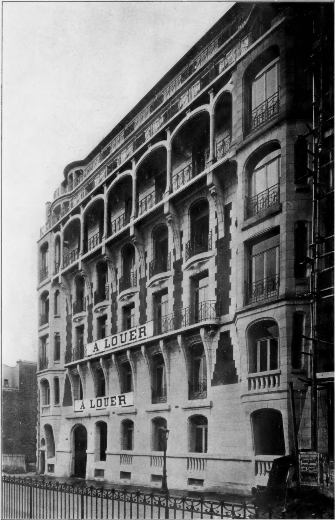
APARTMENT-HOUSE, RUE DE LA TASSE, PARIS, FRANCE.—M. SOREL, ARCHITECT.
