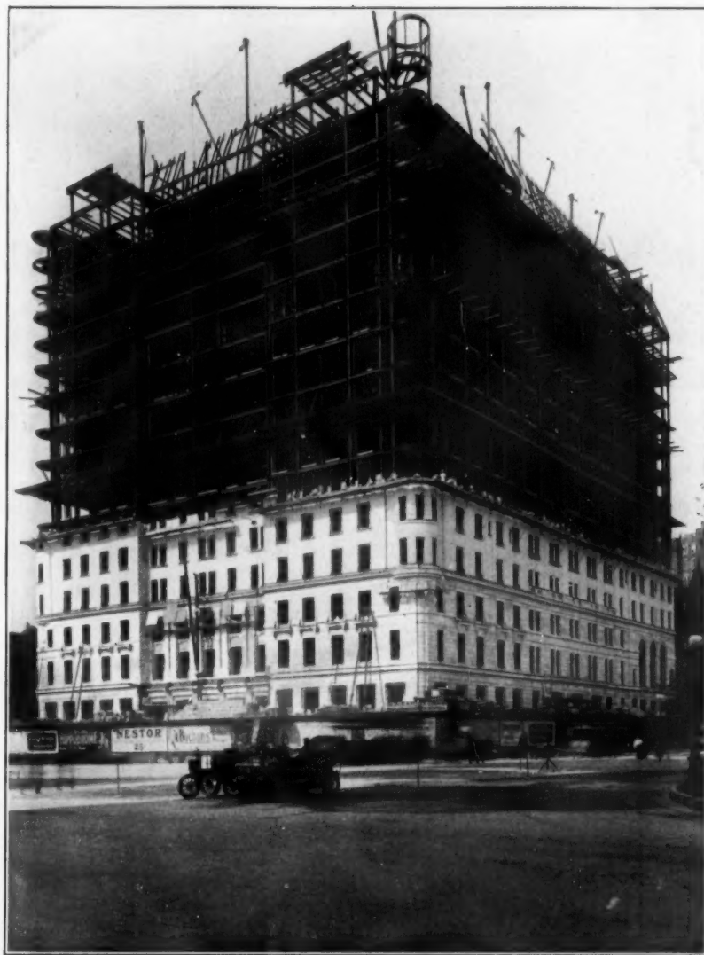
NEW PLAZA HOTEL, NEW YORK CITY STRUCTURAL STEEL PAINTED WITH "SUPERIOR GRAPHITE PAINT"
