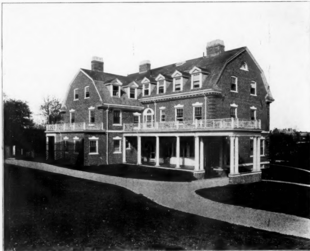
House of J. B. Westbrook, Esq., Brookline, Mass. Chapman & Frazer, Architects.
