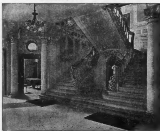
Staircase, American Geographical Society Building
