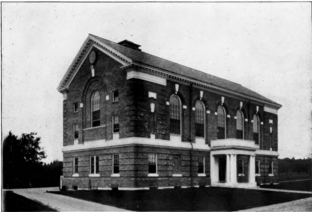
The Dining-Hall: Charles K. Cummings, Architect.
