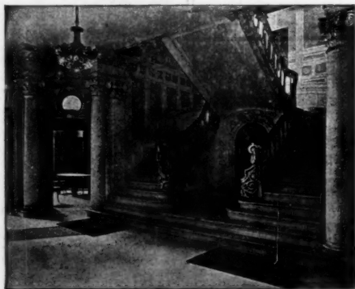
Staircase, American Geographical Society Building
