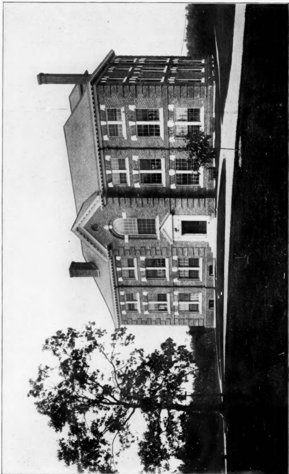
Master's House: Middlesex School, Concord, Mass. Charles K. Cummings, Architect.
