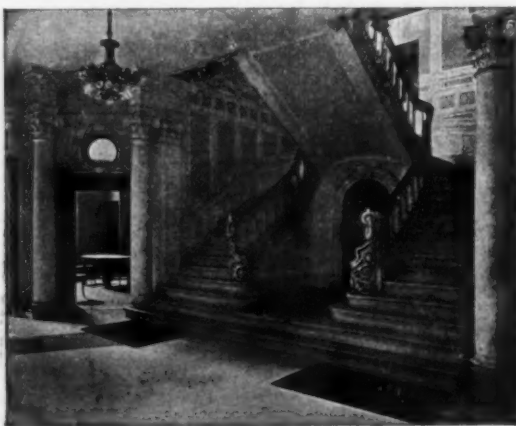
Staircase, American Geographical Society Building
