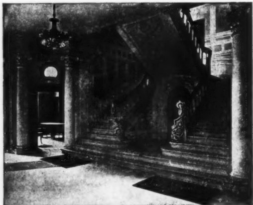
Staircase, American Geographical Society Building
