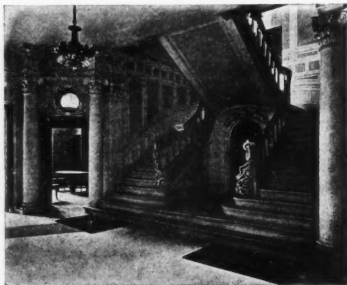
Staircase, American Geographical Society Building
