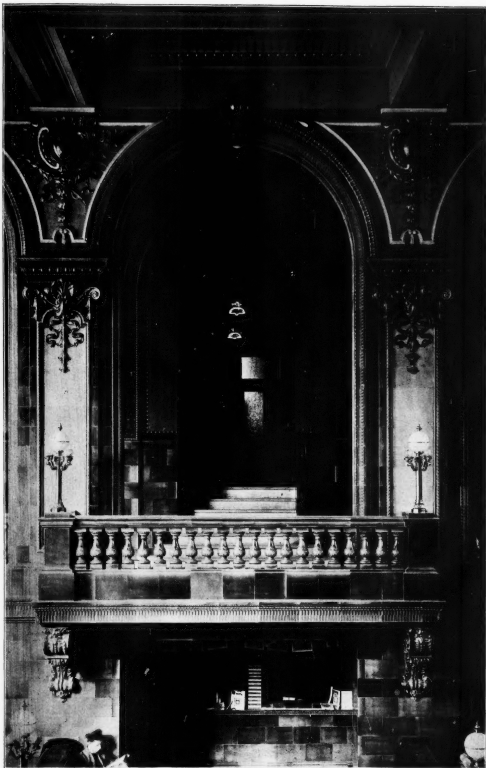
A Bay in the Waiting-room: Union Station, Troy, N. Y. Reed & Stem, Architects.
