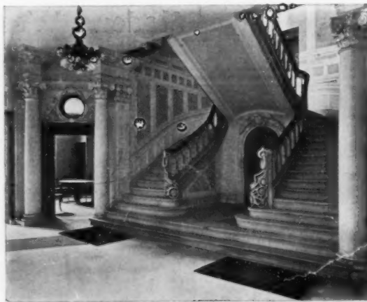
Staircase, American Geographical Society Building
