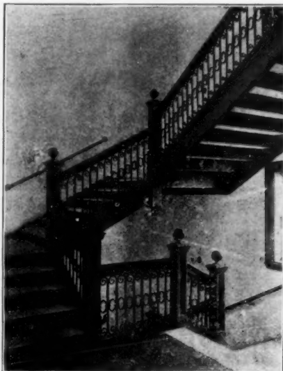
Iron Stairs in the N. E. Conservatory of Music Building Boston, Mass.
