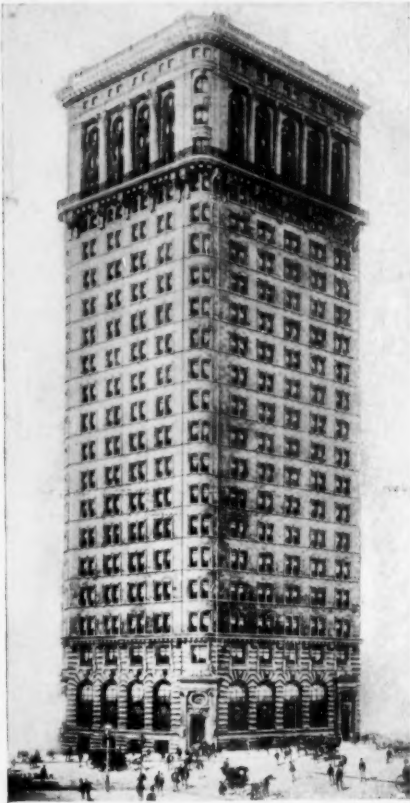
HANOVER BANK BUILDING
