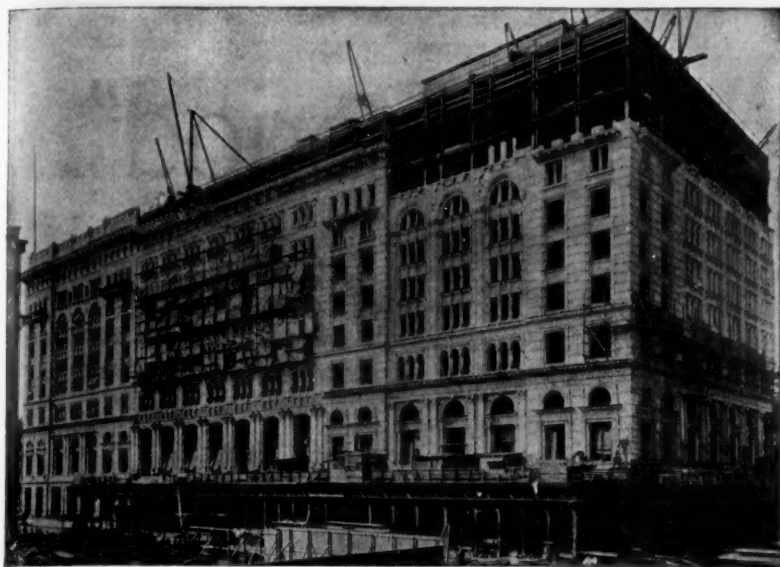
Pearson Flooring Nails are being used throughout on the Metropolitan Life Insurance Building Annex, New York City
