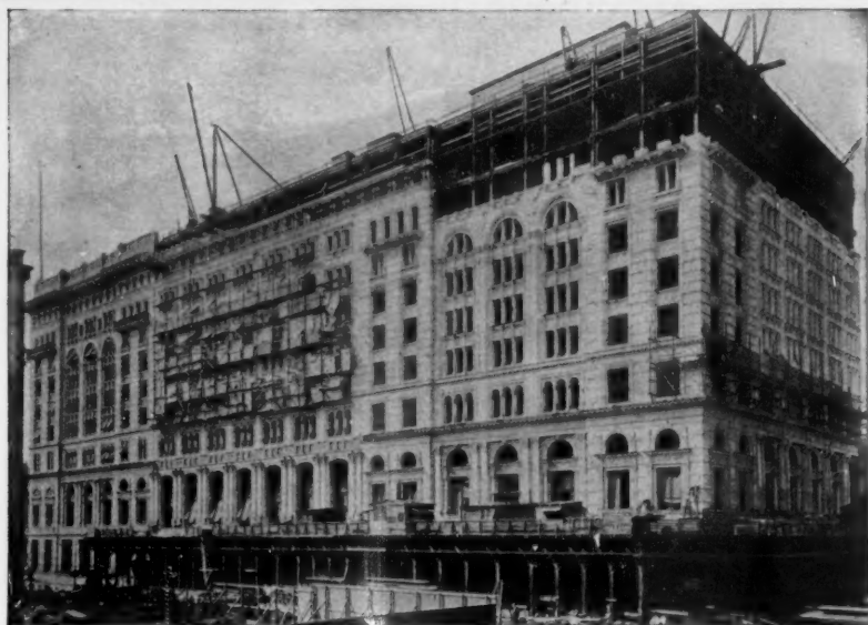
Pearson Flooring Nails are being used throughout on the Metropolitan Life Insurance Building Annex, New York City
