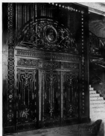
Elevator Enclosure, Hotel Essex, N. Y. City, Howard, Cauldwell & Morgan, Architects
