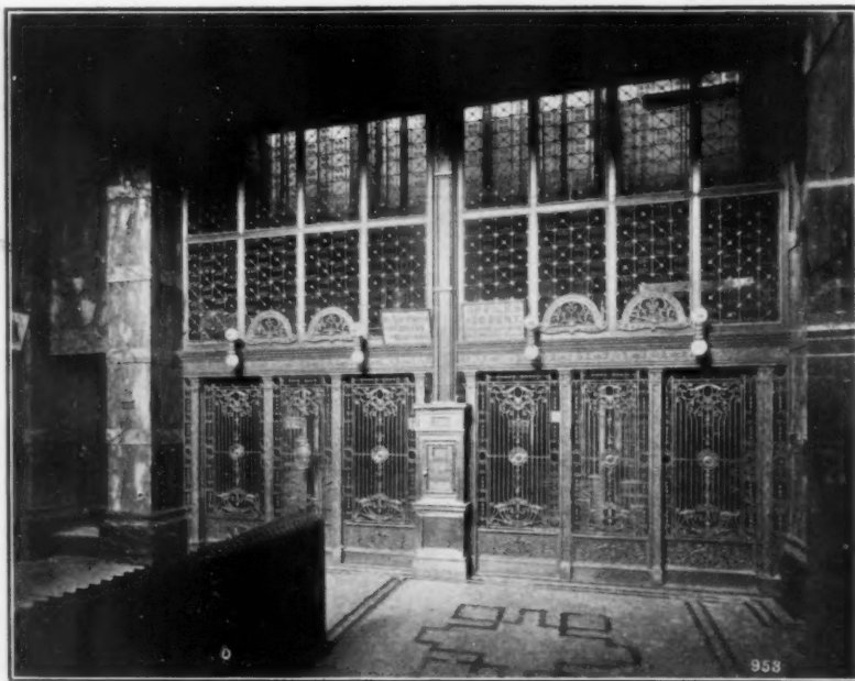
Elevator Enclosures in Rose Building, Cleveland, Ohio
