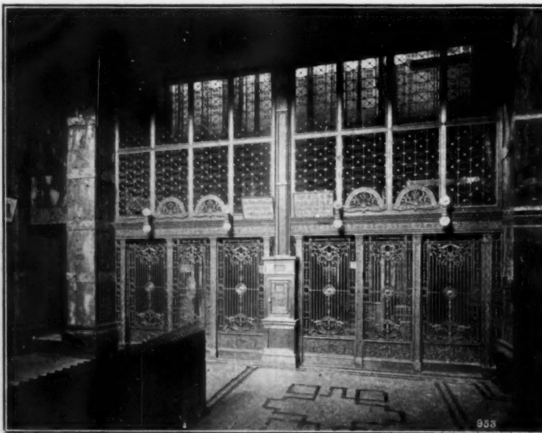
Elevator Enclosures in Rose Building, Cleveland, Ohio
