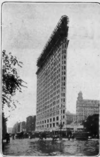
View of the Fuller Building, New York, in course of construction
