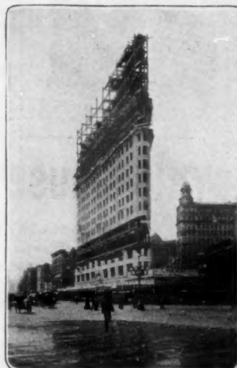
View Fuller Building, New York, in Course of Construction.
