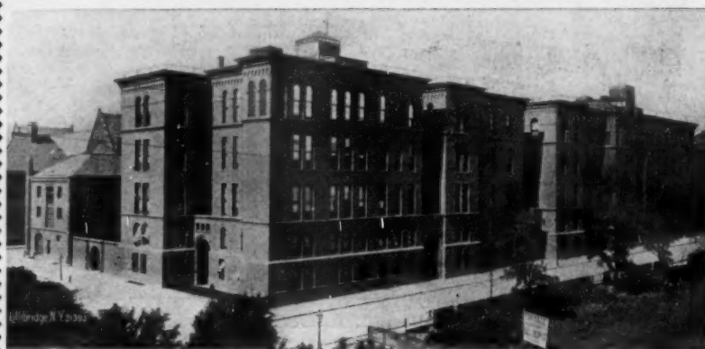
Rear View Presbyterian Hospital, New York City.
