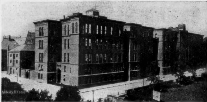
Rear View Presbyterian Hospital, New York City.
