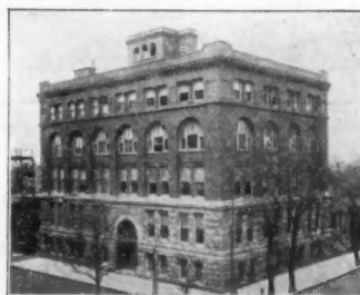
Machinery Hall, Armour Institute of Technology
