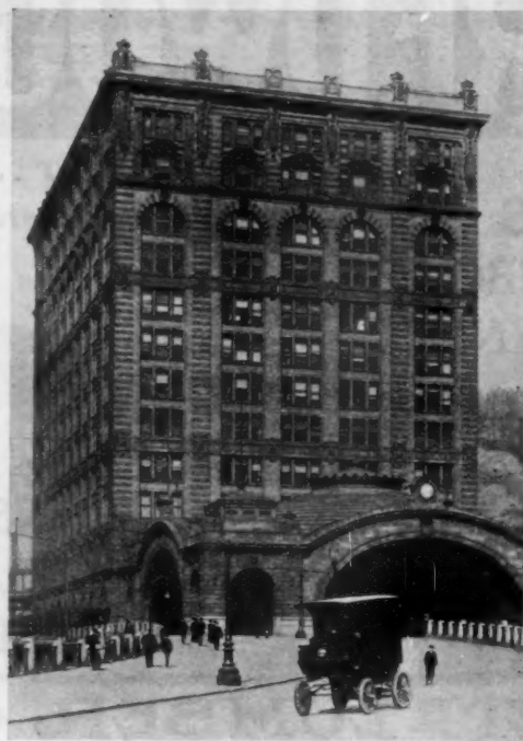
Passenger Station, Pittsburg, Pa. Pennsylvania R. R.
