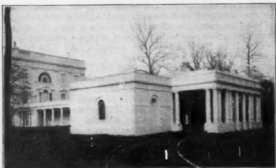
Reception Entrance and East Terrace.
