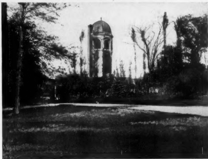
The above Tank Tower contains two tanks of 10,000 gallons capacity each and was erected for a water supply system at Pomfret, Conn., by the Charles J. Jager Co.
