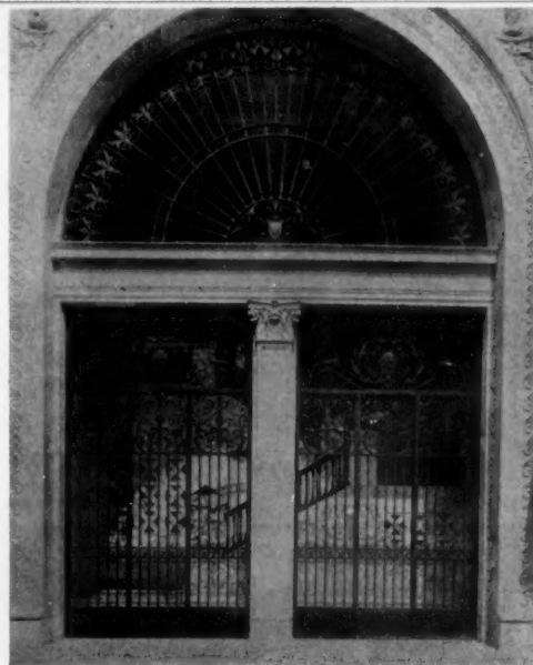
Lyng in Hospital, N. Y. City, R. H. Robertson, Architect.
