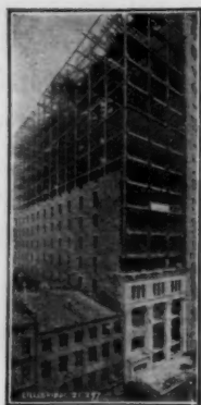
Hudson Building New York
