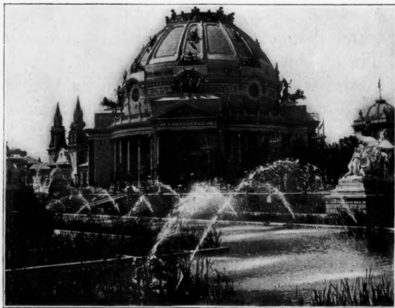
THE ETHNOLOGY BUILDING. GEORGE CARY, ARCHITECT.
