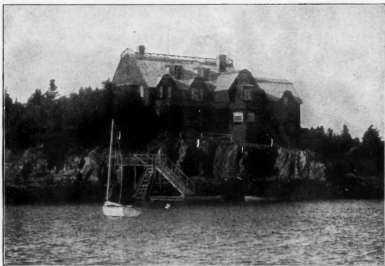
Residence of Dr. Shattuck, Dark Harbor, Me. John Lavallé, Architect, Boston.
