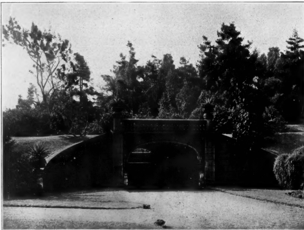
BRIDGE OPPOSITE THE CONSERVATORY, SAN FRANCISCO, CAL.
