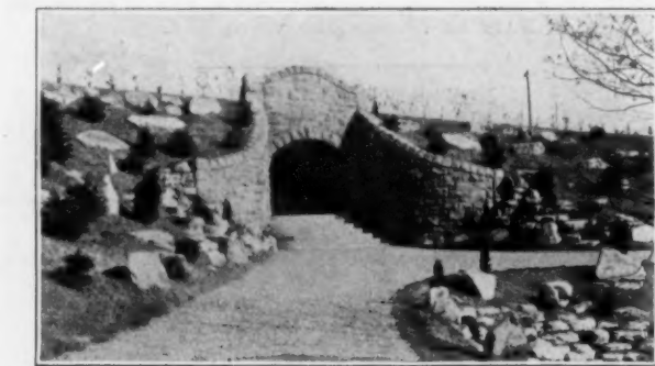
Highland Park, Pittsburgh, Pa., 12' Arch over Footway.
