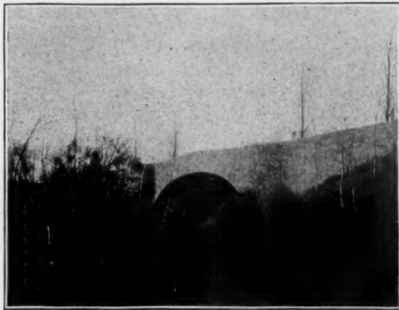
Boylston Bridge, Boston.
