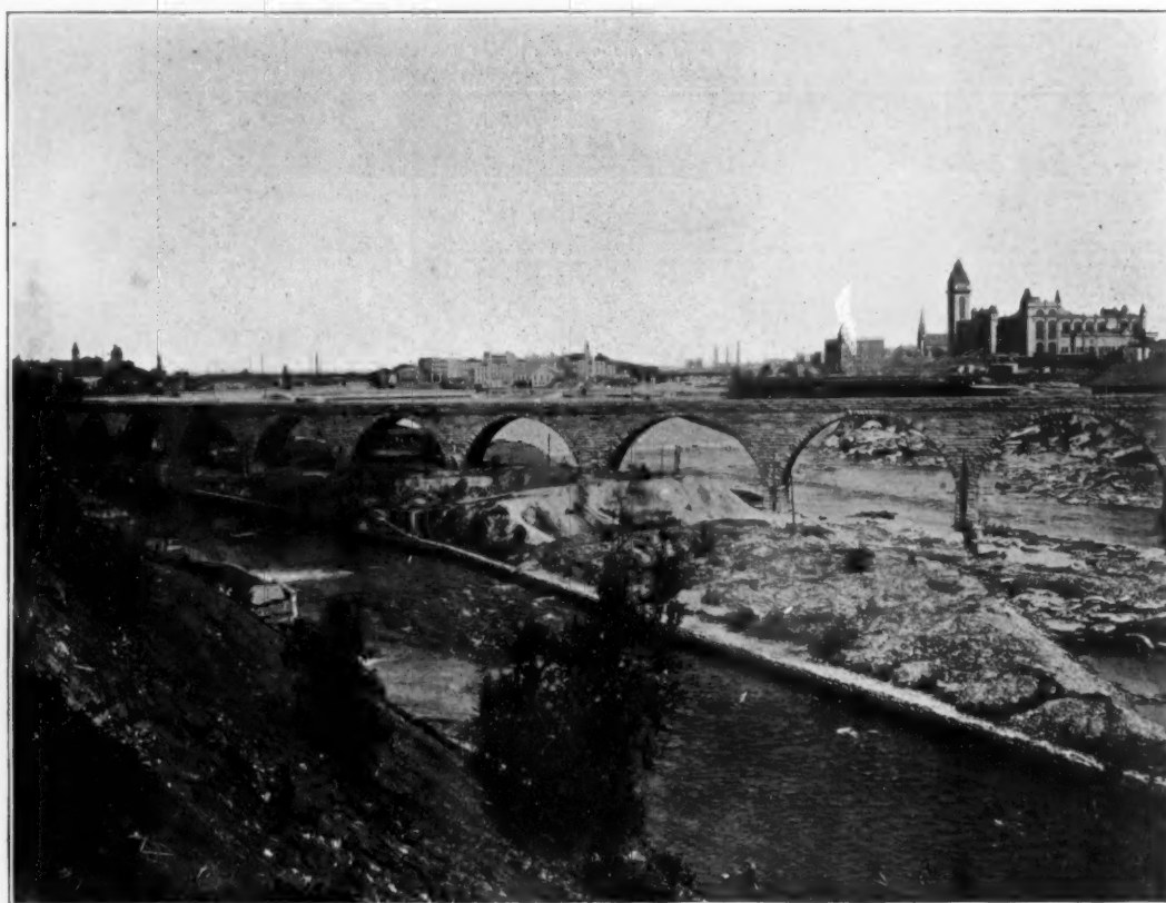
STEEL ARCH BRIDGE AND RAILROAD VIADUCT, MINNEAPOLIS, MINN.
