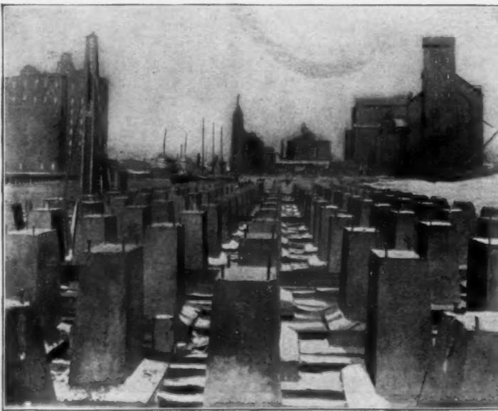
Concrete Foundations, Dakota Elevator, Buffalo, N. Y.
