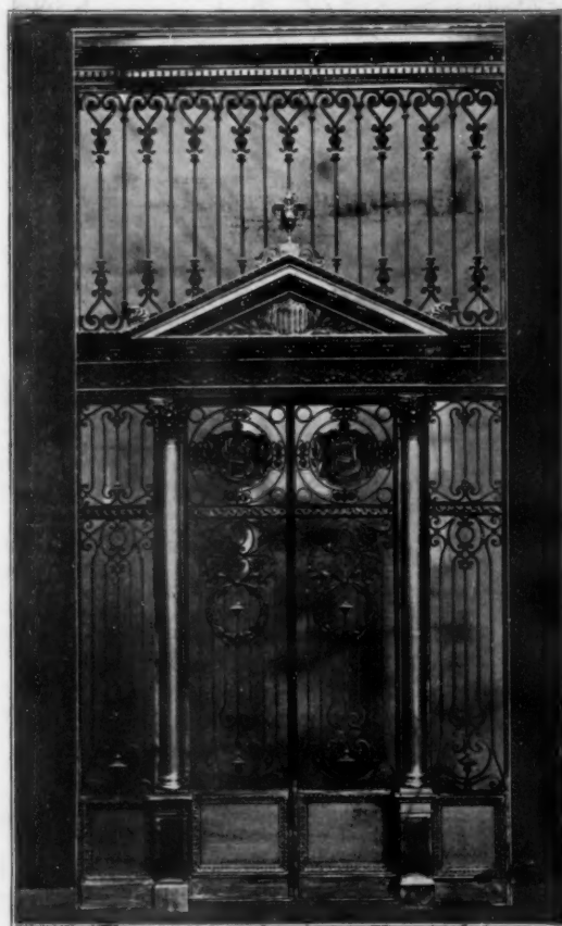
Wrought Iron and Bronze Elevator Enclosures erected in United States Building at Paris Exposition.
