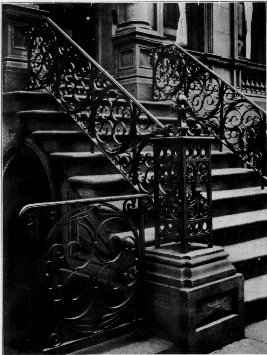
METALWORK XIX.—No. 14 EAST 45TH STREET, NEW YORK, N. Y.
